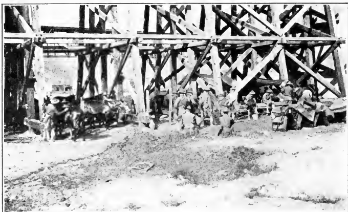
THE CORRAL AT THE CEMENT PLANT
